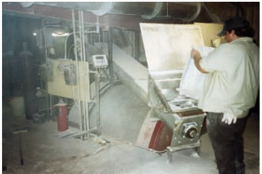
A worker adds 50 pounds of microingredients to the mechanical conveyor's inlet chute, which are then conveyed to the mixer's inlet chute.
